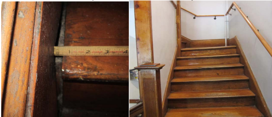
Grand Staircase Problems - Left - City-side Grand Staircase Pulling from Wall Right - Tech-side Staircase is Cockeyed
