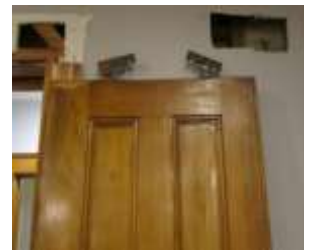
Creative Repairs to the Pocket Doors
