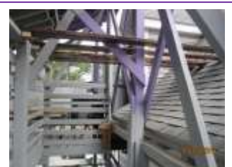
Fixing the Fire Escape
